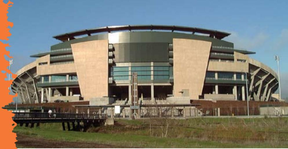
**Architectural Cladding** has become the material of choice wherever low maintenance, economy, strength, and aesthetics are important. Architectural Precast Concrete refers to both the interior structural members and to the exterior facade or “cladding” of a structure. The application of various structural and non-structural shapes, and various finishes, colors and textures, contributes to and enhances the form and finished effect of a building.
